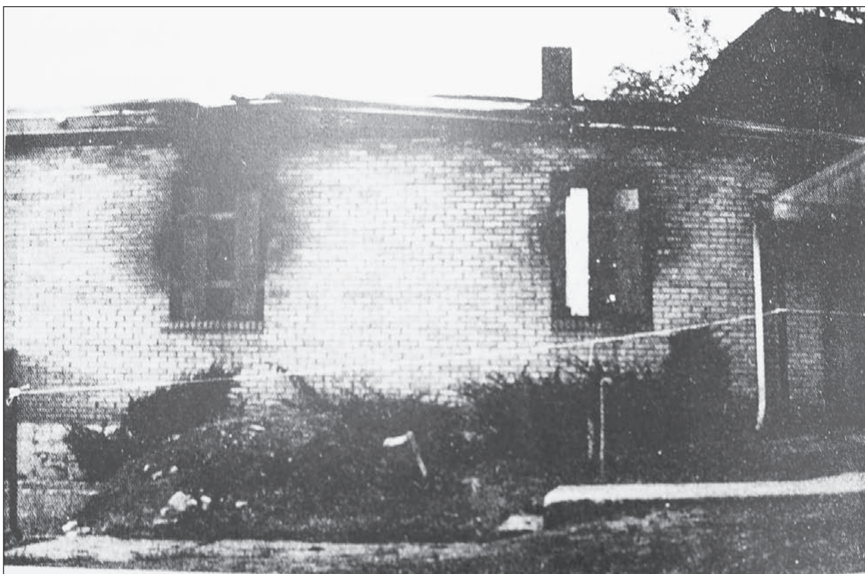
Fire of undetermined origin guts Blessed Sacrament Church Oct. 2, 1974. (Photo provided)
